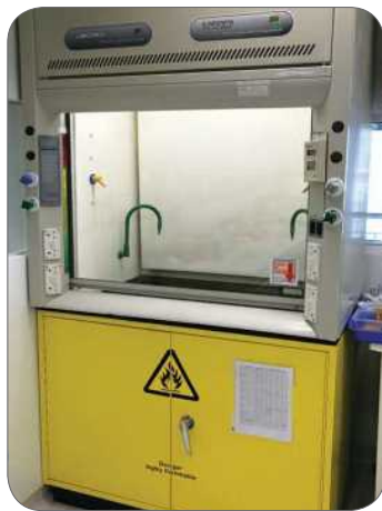
Figure 20: A fume cupboard with a base cabinet specially designed for storage of flammables.
