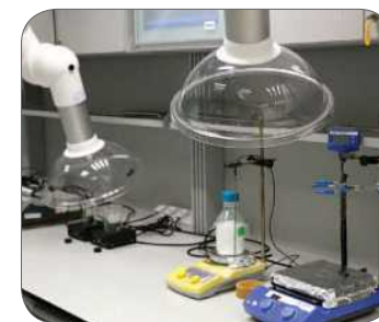
Figure 19: A flexible arm capture hood can be positioned close to the contaminant source.
